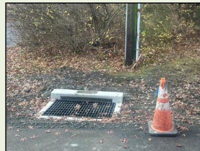
2025 Hill Road Phase I under construction
