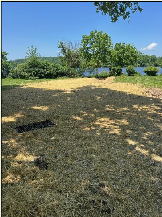
2025 Stormwater Improvement: Three Mile Run Road
