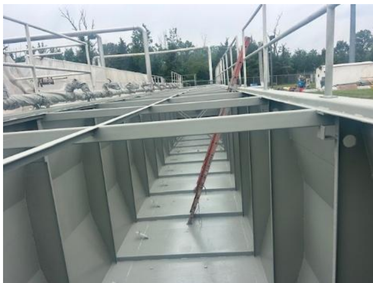
2025 North Aeration Tank Refurbishment
