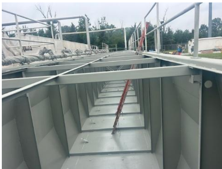
2025 North Aeration Tank Refurbishment
