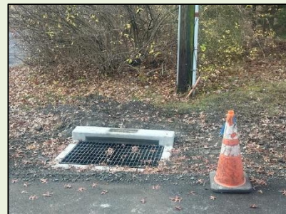
2025 Hill Road Phase I under construction
