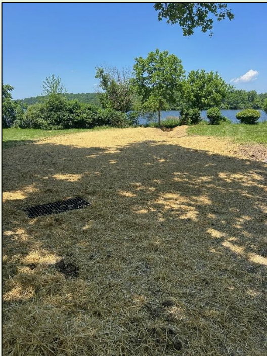
2025 Stormwater Improvement: Three Mile Run Road
