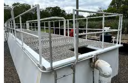
2023 Top of Treatment Tank Repair
