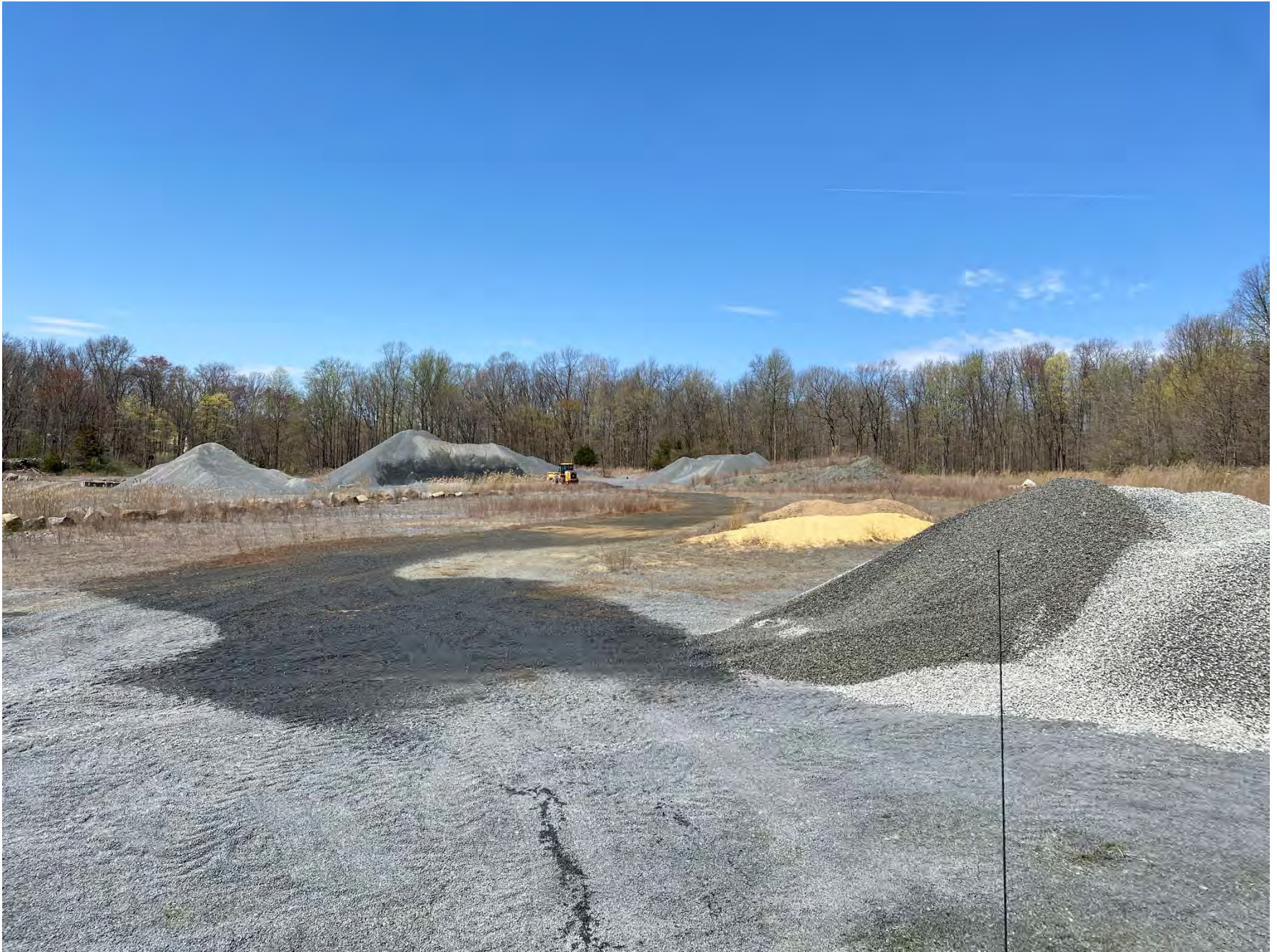
View of wetted crushed stone piles and Rubber Tire Loader travel way
