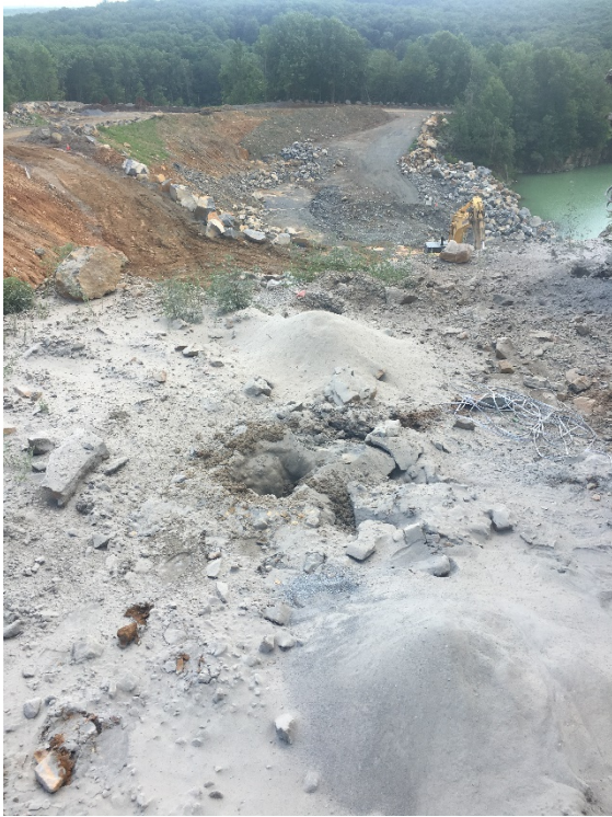
Photo 3 – S-3 Drill Cuttings and Sample Location
