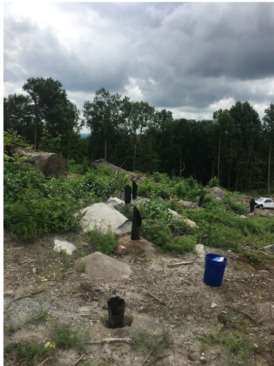
Photo 5 – S-5 and S-6 Drill Cuttings and Sample Locations
