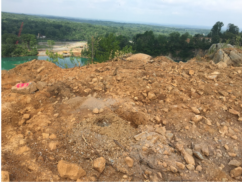
Photo 1 – S-1 Drill Cuttings and Sample Location
