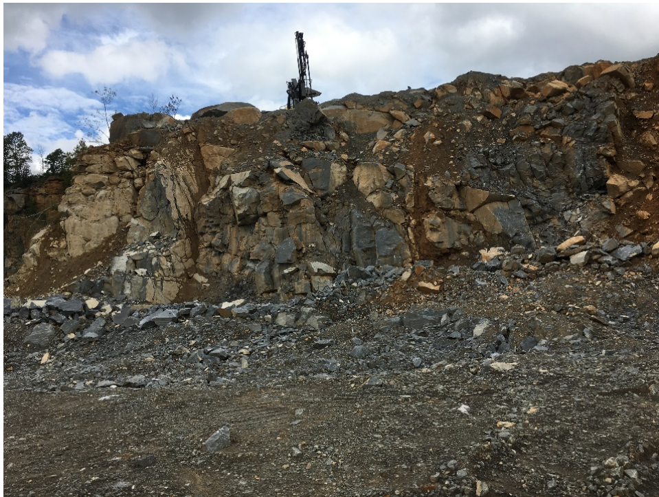
Photo 9 – Highwall of S-11 and S-12 Location
