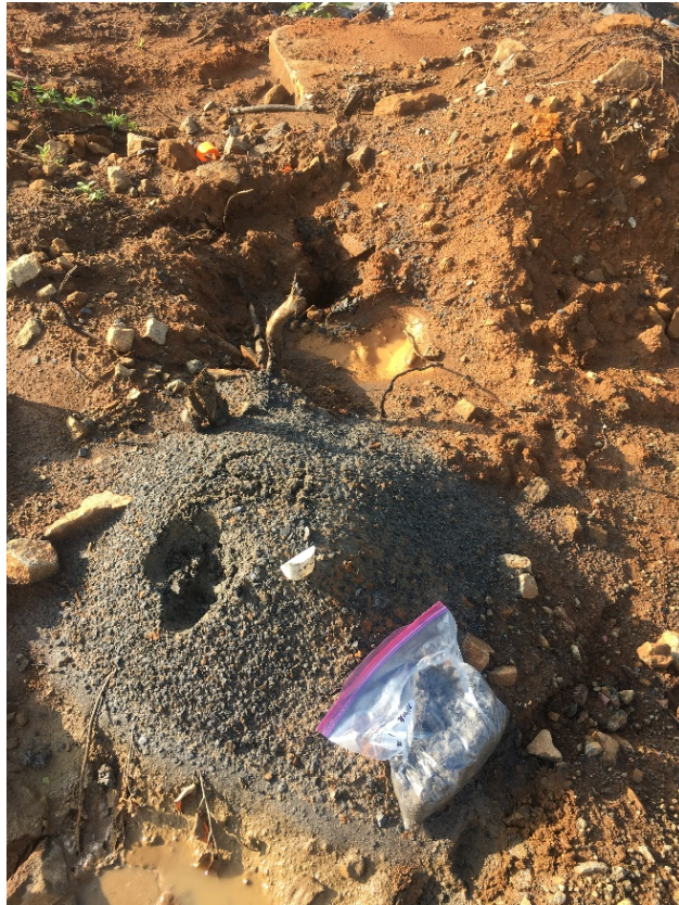
Photo 6 – S-7 Drill Cuttings and Location
