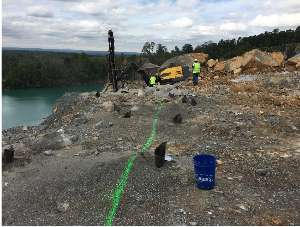
Photo 8 – S-11 and S-12 Drill Cuttings and Locations
